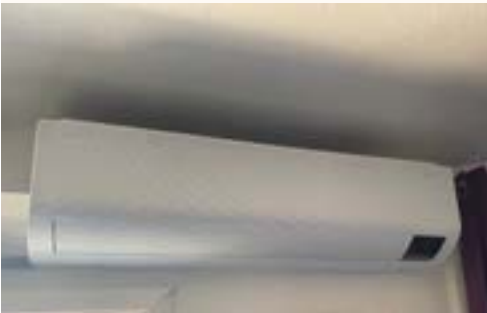
Thermostat (top) and indoor air handler (bottom) for ductless mini-split system.
