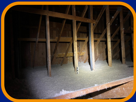
Attic insulation, Sacramento, CA
